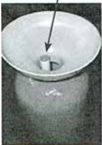
Fig. 1 - The riser (distributor) remains inside the tank seated in the depression at the bottom. The riser should be capped to prevent resin beads from getting inside.
